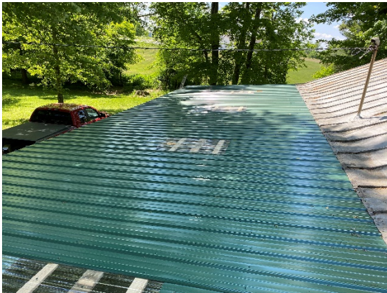
a. New metal roof over the South porch area.
