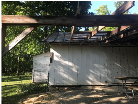
a. New metal roof over the South porch area.
